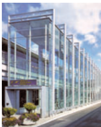
Naaraharju Oy is famous for its excellent steel for welded steel constructions.
