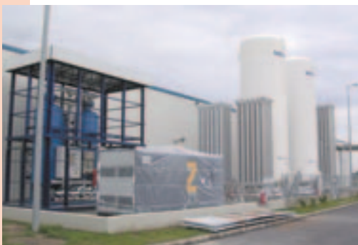
Ibiden, the Japanese manufacturer of diesel particle filters, needs nitrogen and argon for its heat treatment furnaces.
