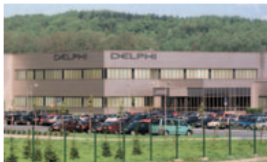
Delphi Polska relies on the use of liquid nitrogen in heat treatment.
