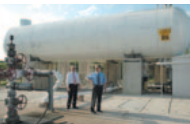
CO 2 is pumped into boreholes in order to increase the amount of oil extracted.
