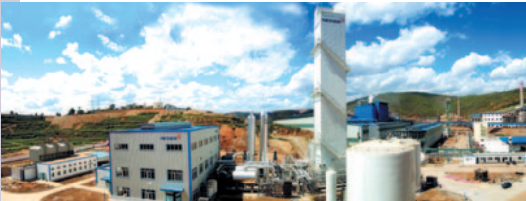
The air separation plant in Yuxi is one of the "prettiest" in the Messer World.
